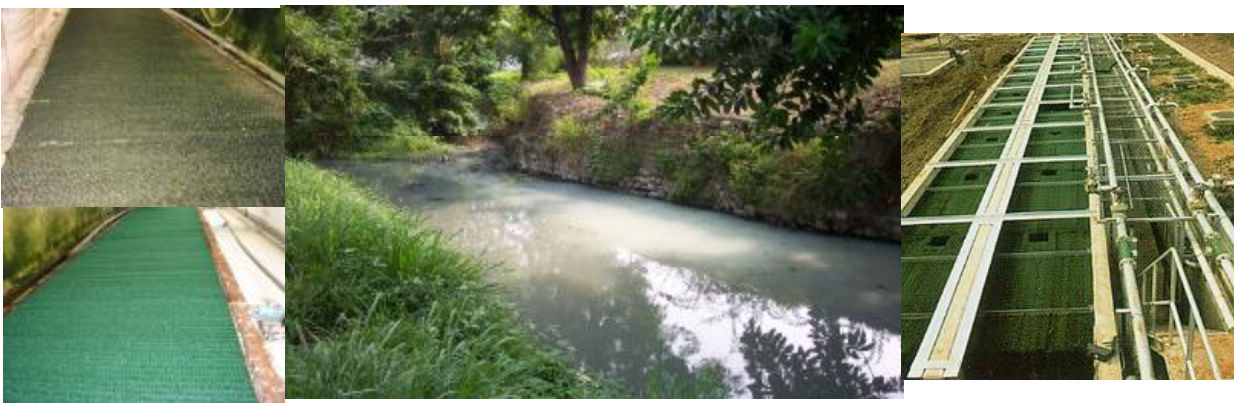
Matala filter media installed in SAF for sewage wastewater treatment (System CE certified)
