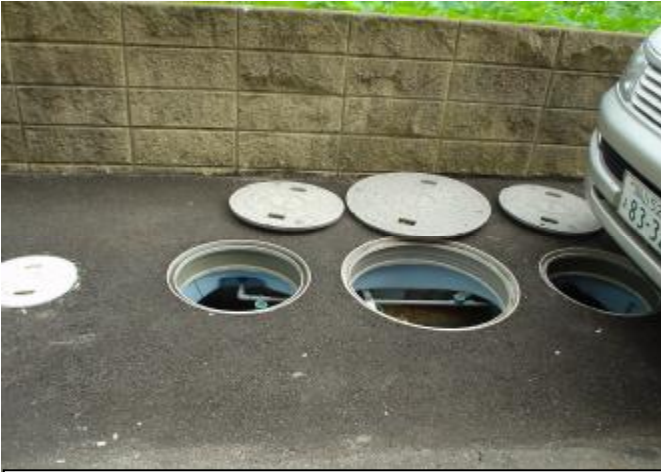
Matala filter media installed in Anerobic chamber for FRP small sewage treatment modul(System licensed in Japan)
