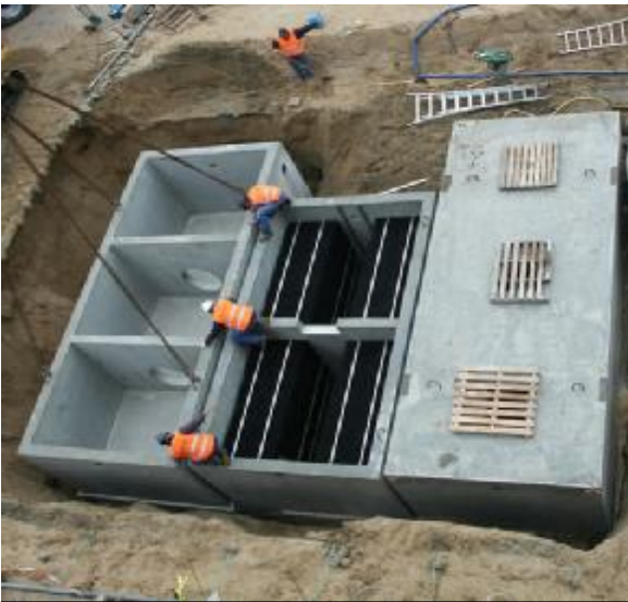
Matala filter media installed in SAF for sewage wastewater treatment (System CE certified)
