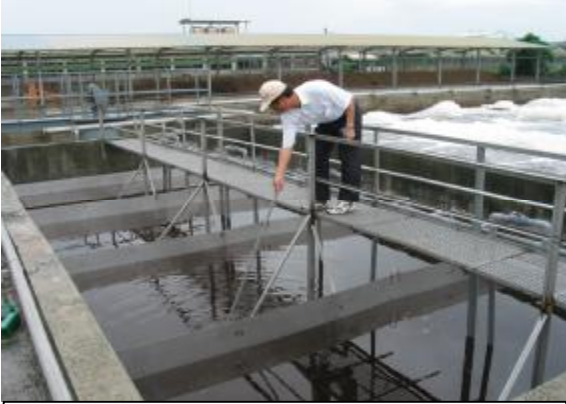
Matala filter media installed as progress biofilter in swine wastewater treatment (- after the Active sludge process)
